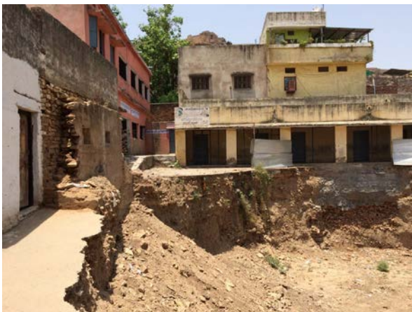
Figure 5. Attempt to stabilize excavation adjacent to nearby school building by applying cement mortar – it is evidently a poorly done job
