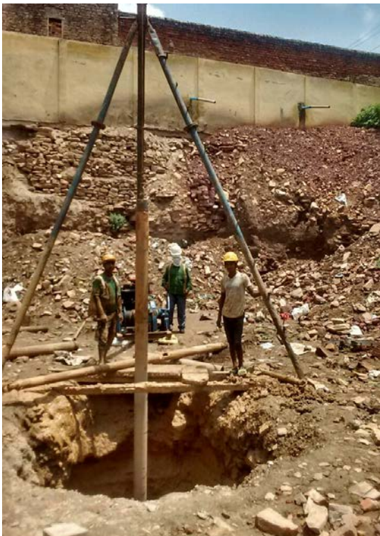
Figure 6. Borehole drilling in progress
