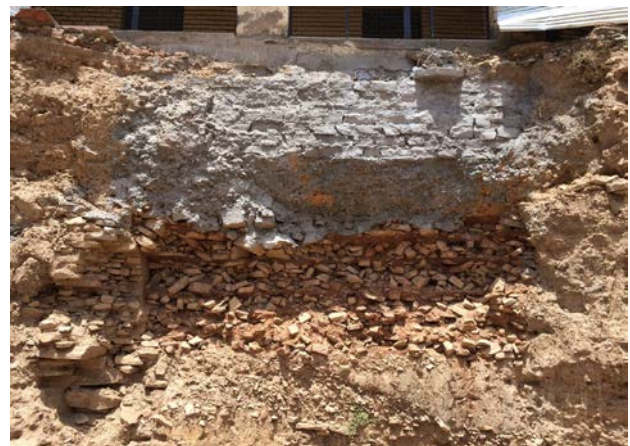
Figure 5. Attempt to stabilize excavation adjacent to nearby school building by applying cement mortar – it is evidently a poorly done job
