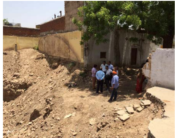
Figure 4. Boulder fill stacked up against wall of existing building
